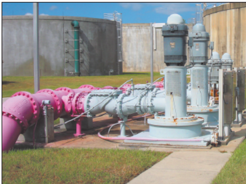
Operating these two 250-horsepower reuse distribution supply pumps at multiple settings on the VFD with slightly lowered pressure overall resulted in water conservation and energy savings that really added up.
